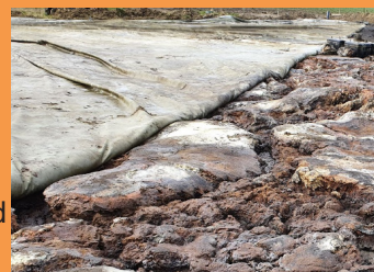
Image showing a floating slurry cover being pulled back after 5 years, crust accounting for 60% of storage volume
